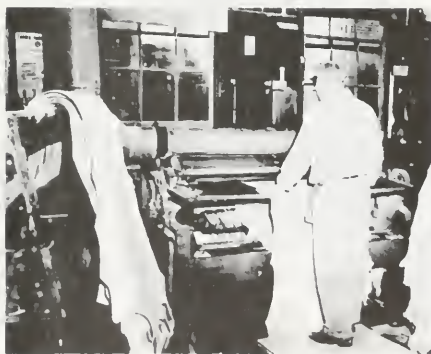
14 Smoothing the grain surface of side leather on a buffing machine.
